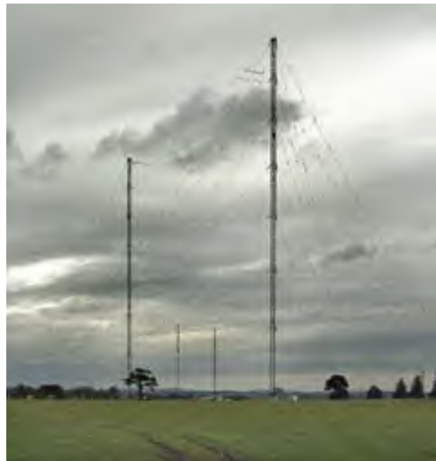
Droitwich transmitter currently radiates BBC Radio 4 with 500 kW on 198 kHz from the T-antenna strung between two 700 ft guyed masts. [Credit: Bob Nienhuis, released to public domain.]
