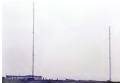
BBC MF transmitting site at Moorside Edge, midway between Leeds and Manchester in northern England. [1982 G3VNO pic.]
