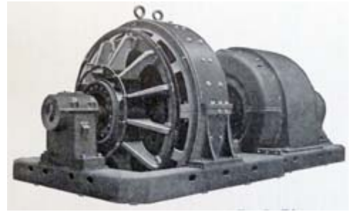
DC generator driven by an AC synchronous motor. [Metropolitan Vickers, Manchester.]
