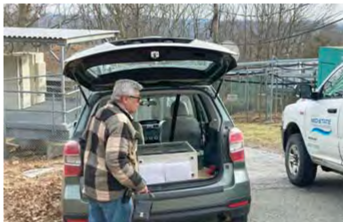
Bob prepares to install the MTR3000 at the repeater site.
