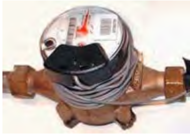
Neptune T10 water meter register installed in 2004. Note gray wire to meter interface unit.
