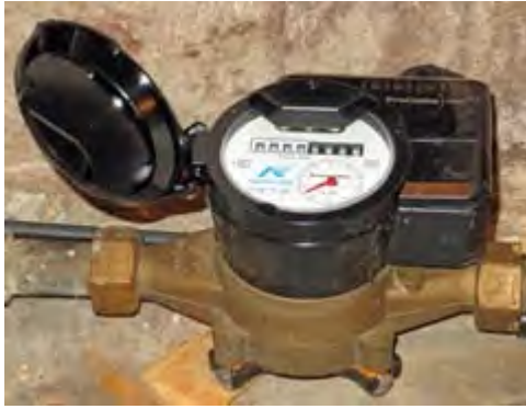
The mechanical register can be read manually by opening the hinged plastic cover.
