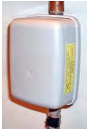
Neptune R900-v2 Meter Interface Unit transmitted water data in the range 910-920 MHz
