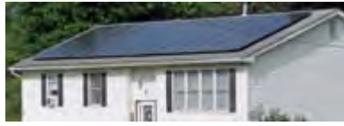
Roof-mounted solar cells.
