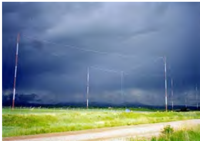
Photo of the four 400 ft towers supporting one of the twin antennas for WWVB. Top-loading wires and radiating downlead have been emphasized for clarity. [Credit: NIST.]
