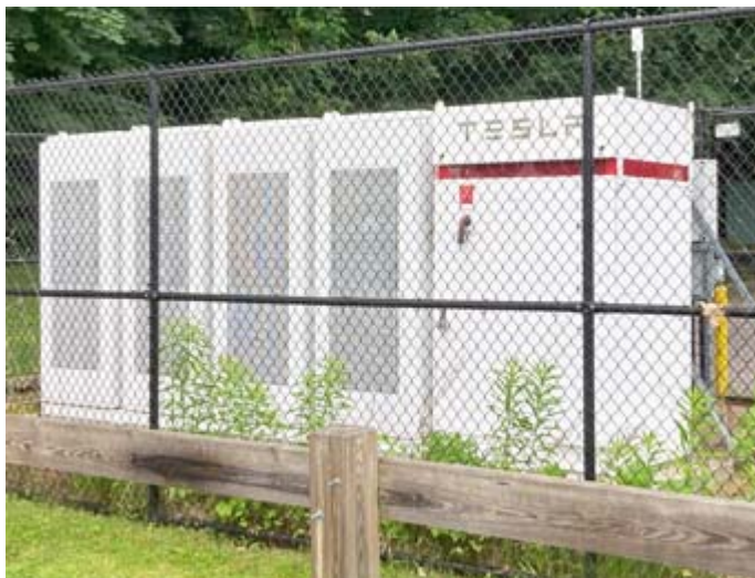
490 kW Tesla Powerpack battery energy storage system in use at Staples Plaza, Yorktown Heights uses lithium-ion cells to store energy from the rooftop solar array. Sodium-ion could provide a safer technology for future static installations.
