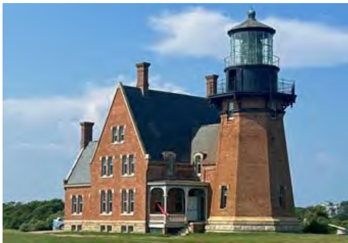
Block Island Southeast Lighthouse, New Shoreham RI.
