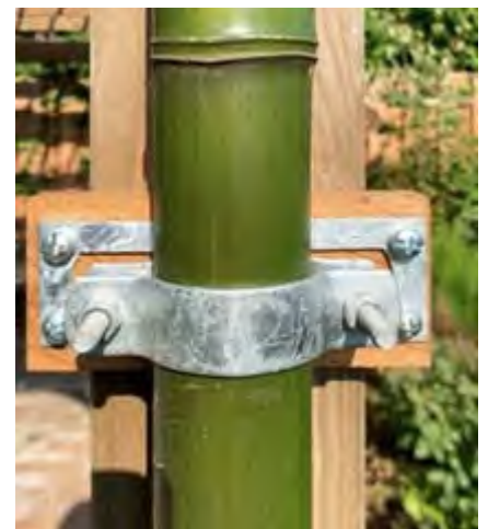
Treated bamboo pole as antenna support. [Photos credit:WA4ARB].
