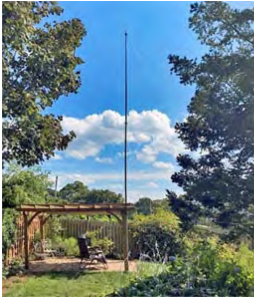
Guyed mast made out of a 35 foot bamboo pole is fastened to the pergola for support.
