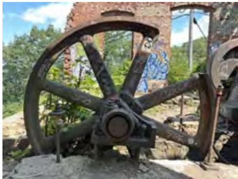
Wheel House near northern summit of Mount Beacon hauled tourists to the former Hotel and Casino.
